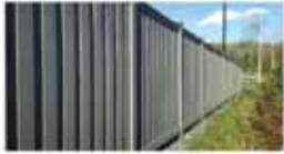
COMPOSITE FENCE (AT-GRADE OR TPSS)
