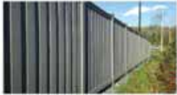
COMPOSITE FENCE (AT-GRADE OR TPSS)
